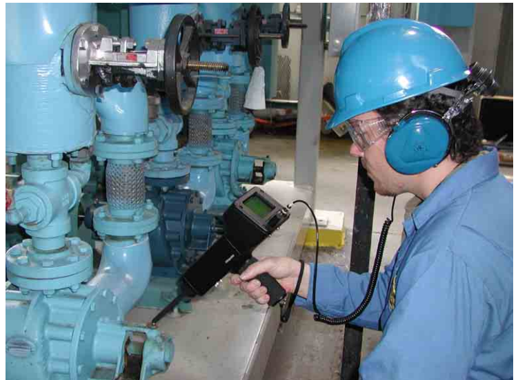
Figure 1. UE Systems ultrasonic detector hears if a bearing is malfunctioning; Photo courtesy of UE Systems Inc.
